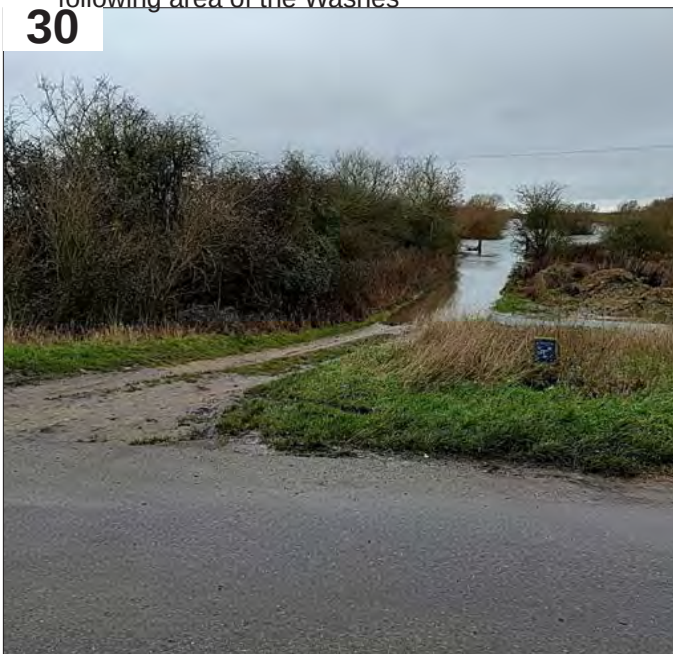
30: Access onto the washland
