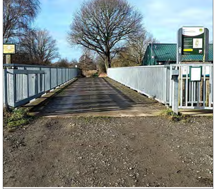
1b: Bridge onto the site and information signage
