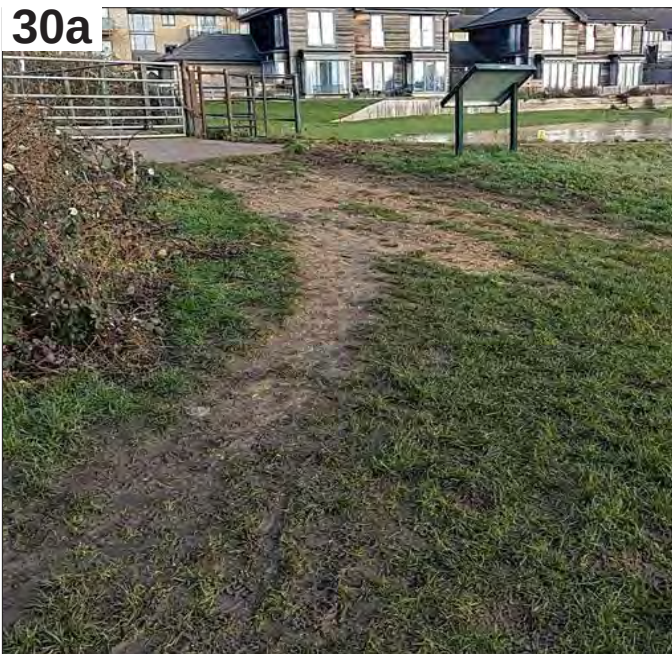
30a: Footpath erosion at entrance to Portholme Meadow
