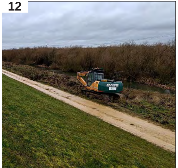
12: EA heavy machinery parked on the track parallel to the River Delph
