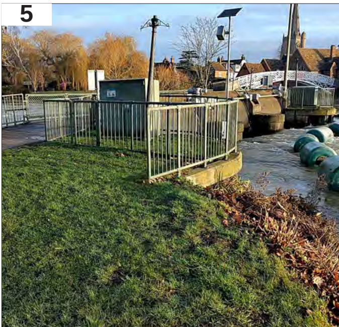
5: Bridge and sluice over Great River Ouse
