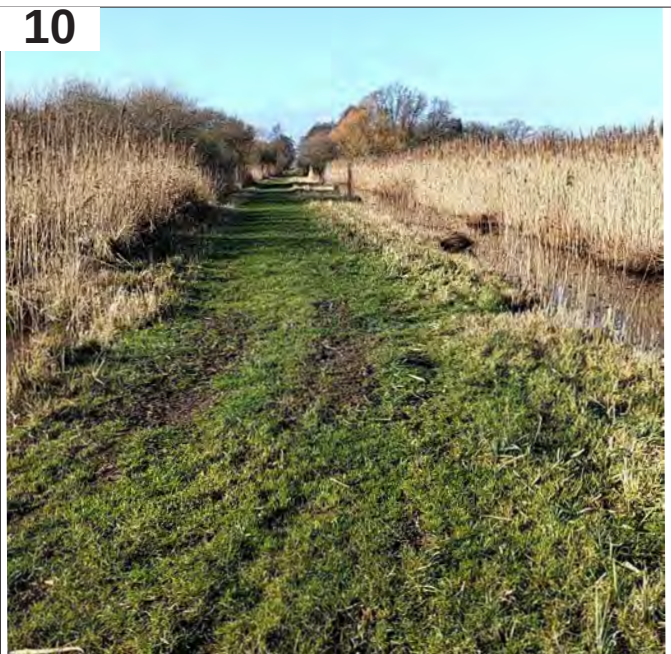
10: Light vehicular erosion of managed route around site
