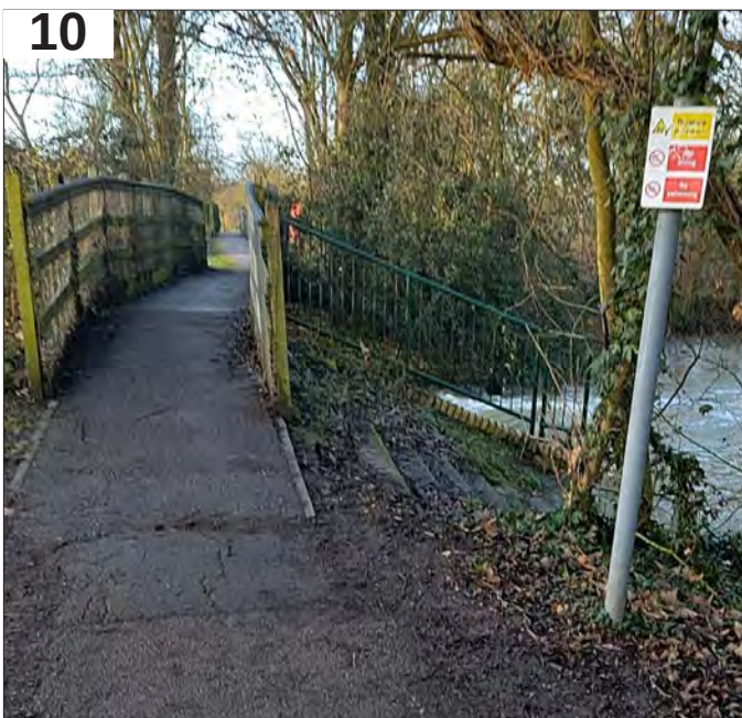
10: Bridge and no swimming sign
