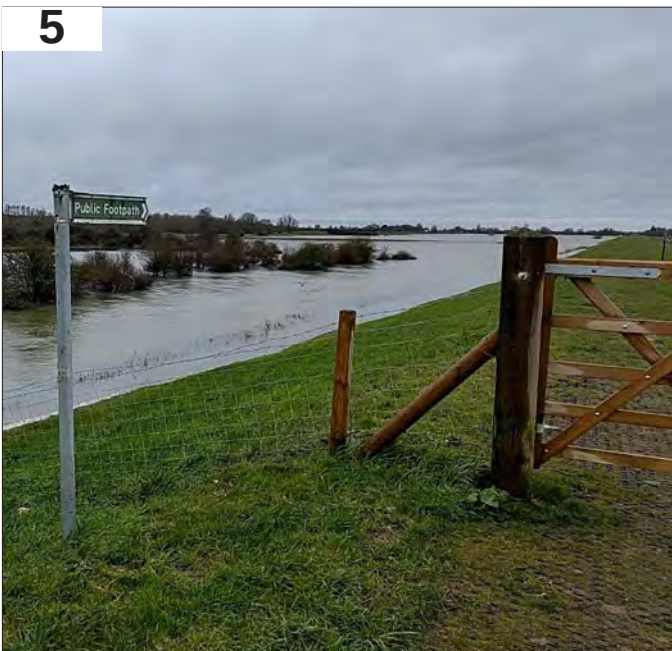
5: Signage and gating of the PRow
