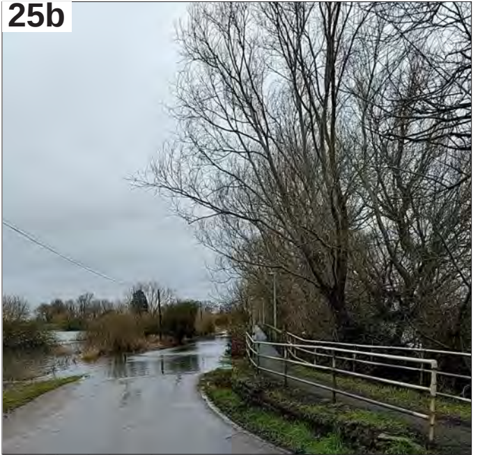
25b: Flooded road access and pedestrian walkway
