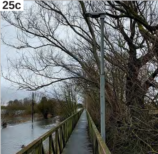
25c: Pedestrian raised walkway and lighting
