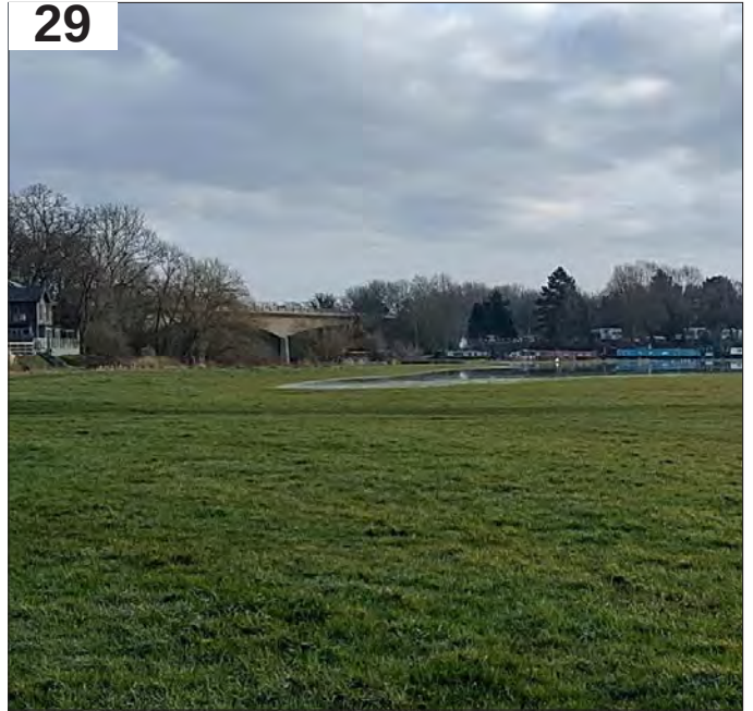
29: Exposed A1307 bridge over the River Great Ouse
