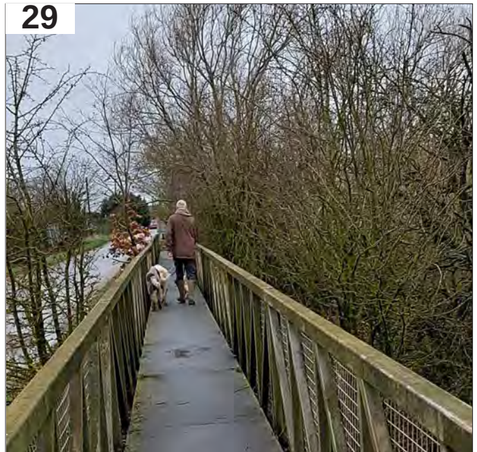
29: Dog walker utilising raised pedestrian walkway
